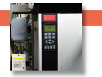
These systems are often designed in such a way that fans run at a constant speed, with their output controlled downstream by a mechanical valve. It's much more efficient to control the speed of the fan itself using a VFD.
